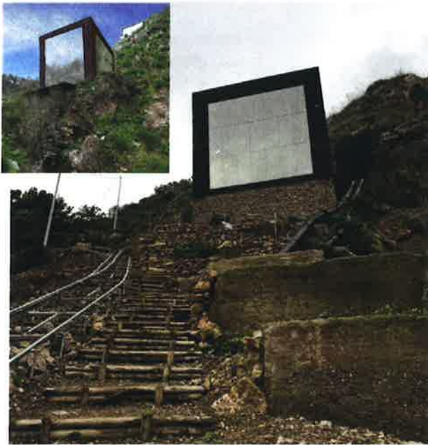
Centrale Alcantara 1 – Post Operam
